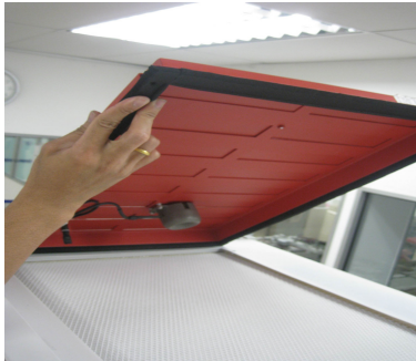
Figure 5.7. Lifting & Removing the Damper
