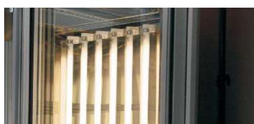
FIT D - light tubes installed in door
