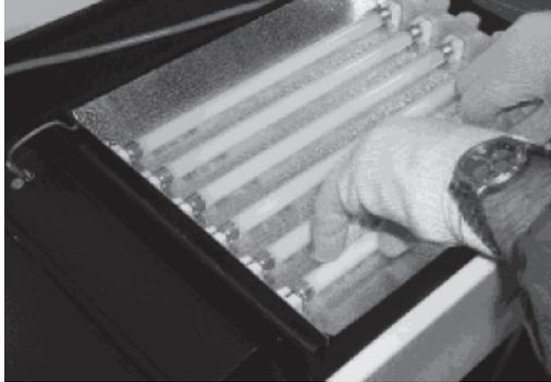
7. Remove the lamp. Install the new lamp by rotating it so that the pins are horizontal and the lamp is tight.
